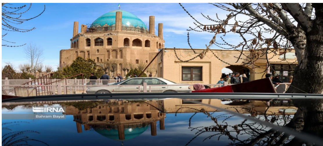
Figure 2: An overview of the historic Dome of Soltaniyeh structure
